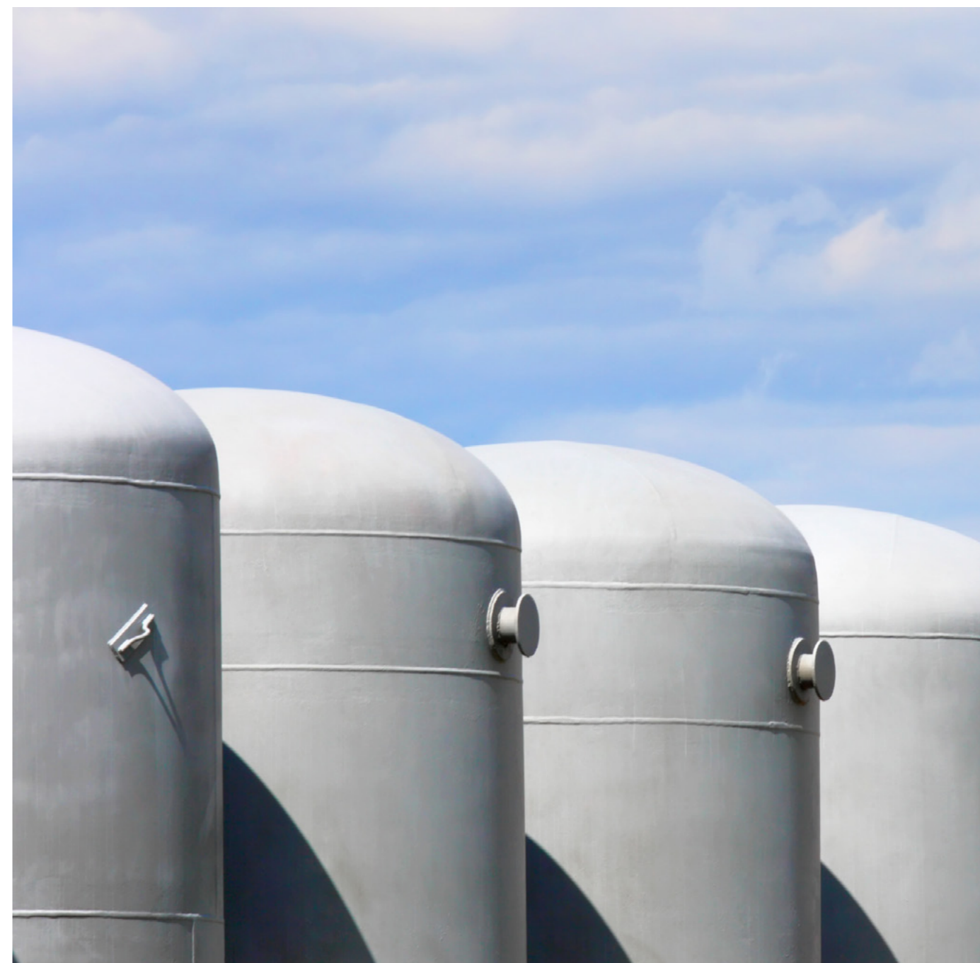
↑ Storage in compressed tanks is beneficial for optimising production over a few hours and days. In regions with high share of solar PV in the mix, such as in Chile, the price difference during the day is expected to incentivise flexible hydrogen production during daytime combined with short-term storage.
